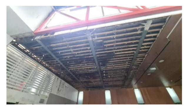
The First Floor level the Counselling Room ceiling is not exhibiting fire damage to structure, the area of fire damage is again localised there around the double height glazed void which extends up to the roof terrace level. Again the surrounding rooms were observed to be in better condition than expected.
