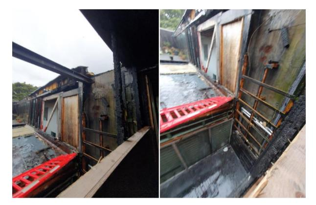
In areas where there is localised severe fire damage, the design team have recommended the removal of these roof sections with charred structural joists for health and safety reasons. They have also recommended the installation of waterproofing works to ensure areas that are in relatively good condition do not deteriorate. These works will be undertaken in the coming weeks and will reduce the scope of the main repair and reinstatement works.
