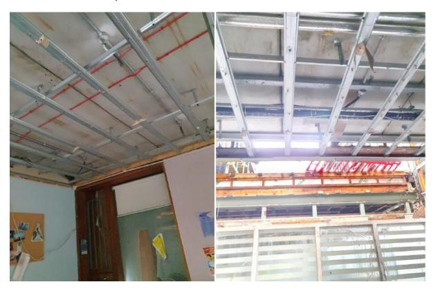
On the Second Floor level there is severe fire damage to the double height void at roof terrace. Fortunately the other rooms surrounding this zone appear to have sustained lesser fire damage in comparison. The Meditation room fire damage is localized to the glazed envelope and the side facing the stairs.
